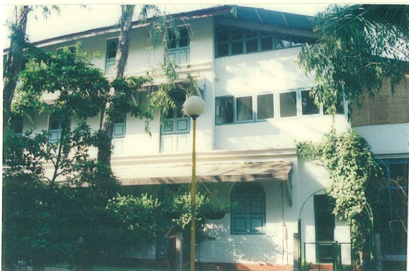
Side view showing extension at the back
