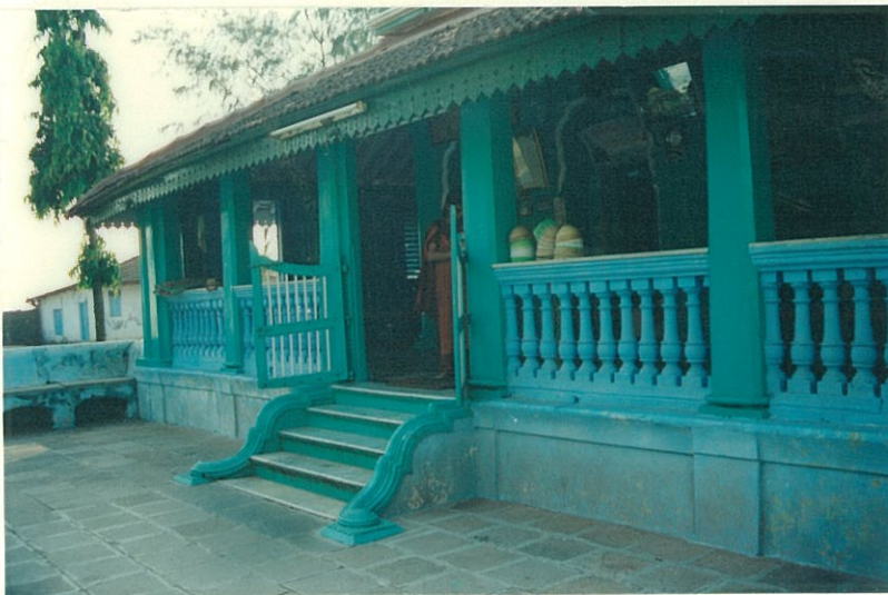
Steps from the front court lead to the timber frame verandah surrounding the tomb chamber
