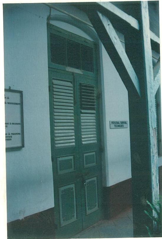
Door detail showing movable wooden louvers
