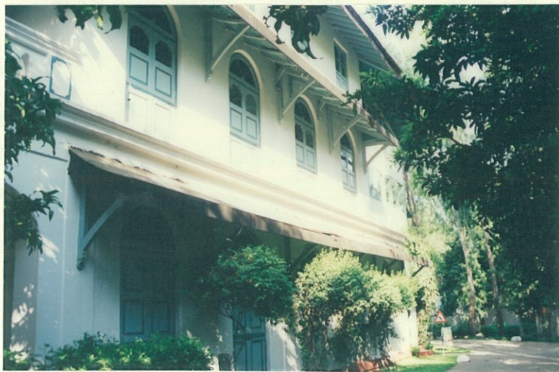
Side view showing a running, deeply overhanging chhajja
