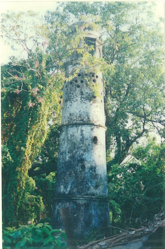
Corner minaret, one in each corner of the square tank
