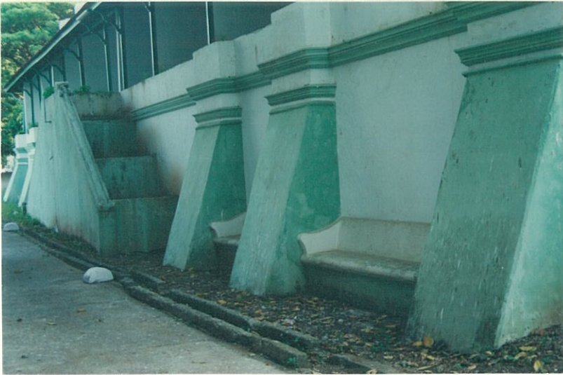
Built in seats between the buttresses, facing the sea
