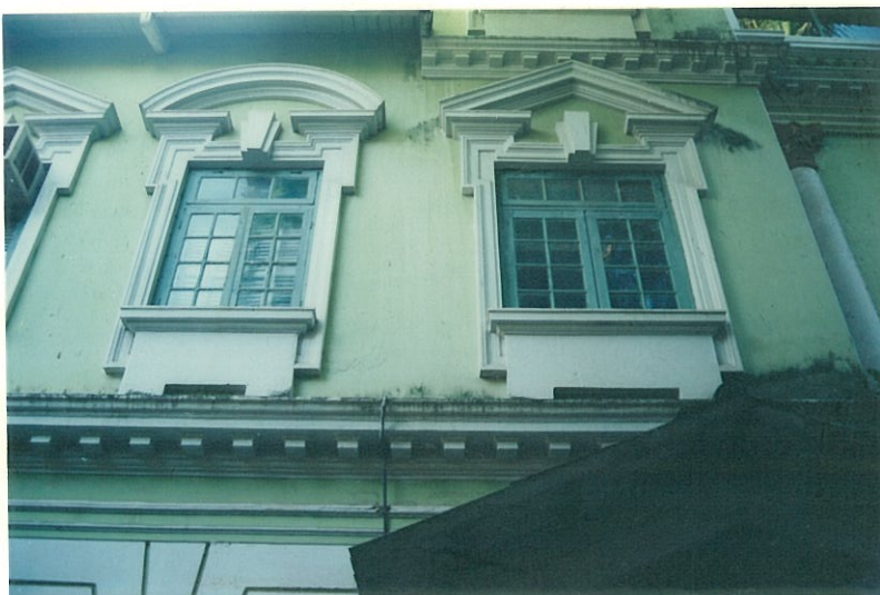
Windows with highlighted stucco mouldings with broken pediments and exaggerated key stones
